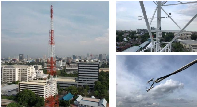
Figure 1 Eddy covariance system at the KU tower
